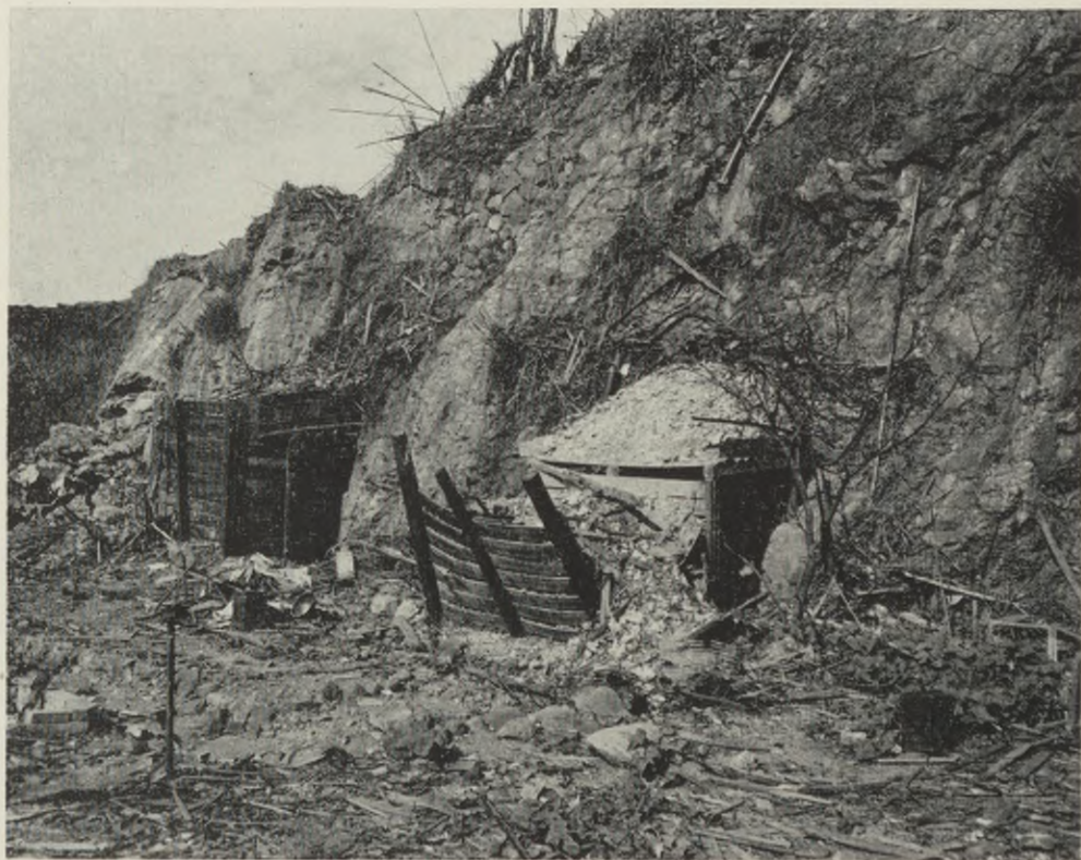
Photo 36. Pictures showing conditions of tunnel shelter entrances located 35 to 50 yards from the center of impact of the atomic bomb.
